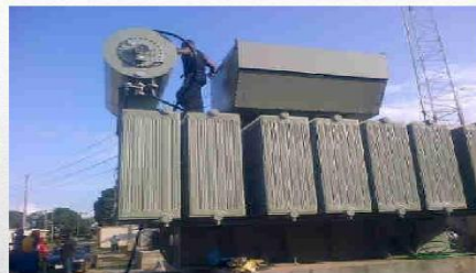
Construction, Installation and Commissioning of 15 MVA Transformer at the Eagle Island Injection Sub-Station in Port Harcourt, Nigeria, by Sigma
