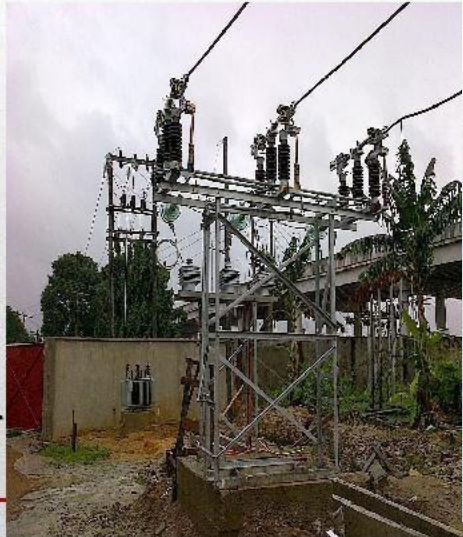
Sigma Engineer Installing Gantries for Ministry of Works 15 MVA Injection Sub-Station at School of Nursing Site, Port Harcourt, Nigeria
