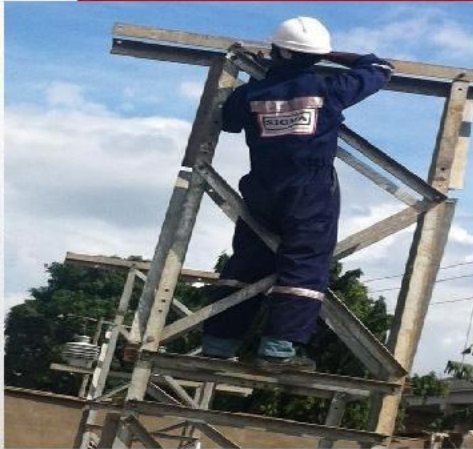
Sigma Engineer Installing Gantries for Ministry of Works 15 MVA Injection Sub-Station at School of Nursing Site, Port Harcourt, Nigeria
